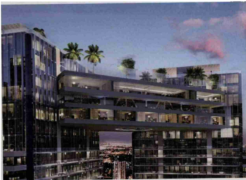
ABOVE: One River Point's sky bridge will link its two towers and house the private members-only 35,000-square-foot Sky Club.
